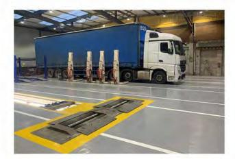
In order to meet the stringent Health and Safety standards required, PSC masked out and laid 100mm edging lines in Resdev Pumatect V high build epoxy resin, safety yellow around 3 HGV pits, shaker plates and rolling roads totalling 104 linear metres. As an additional measure further 75mm wide epoxy resin demarcation lines in white were laid to aid reversing the HGV vehicles.
